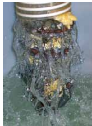
4" CHEESE PRODUCTION PIPELINE
