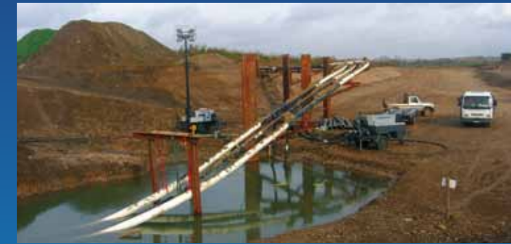
6" OXYGEN PIPELINE (CLEANING, TESTING, DEWATERING AND DRYING)
