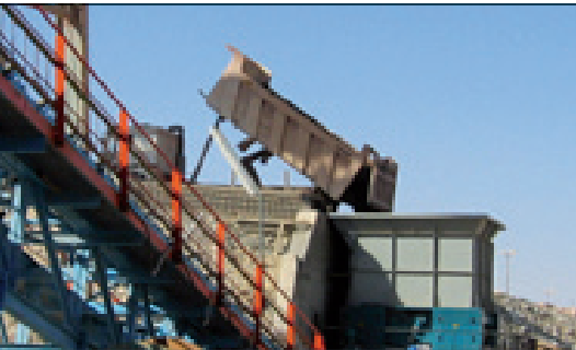
TRANSFER OF OIL EMULSIVE SOIL OR PLASTIC WASTE FROM A TRUCK Hopper with OSZILLOMAT discharge. Place: Egypt
