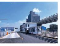
Overview: Ensa invests, constructs, and operates projects. The project adopts a continuous counter-current water washing, thermal mercury removal & MVR process. Fly ash undergoes dechlorination and mercury removal to obtain some industrial raw material products, and the residue enters the cement kiln system for resource utilization and disposal.
