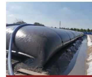
土工管袋脱水 Dewatering of Geotextile Bag
